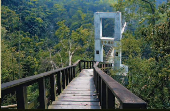
瑞里青年嶺吊橋 Rueili: Cingnian Peak Suspension Bridge
