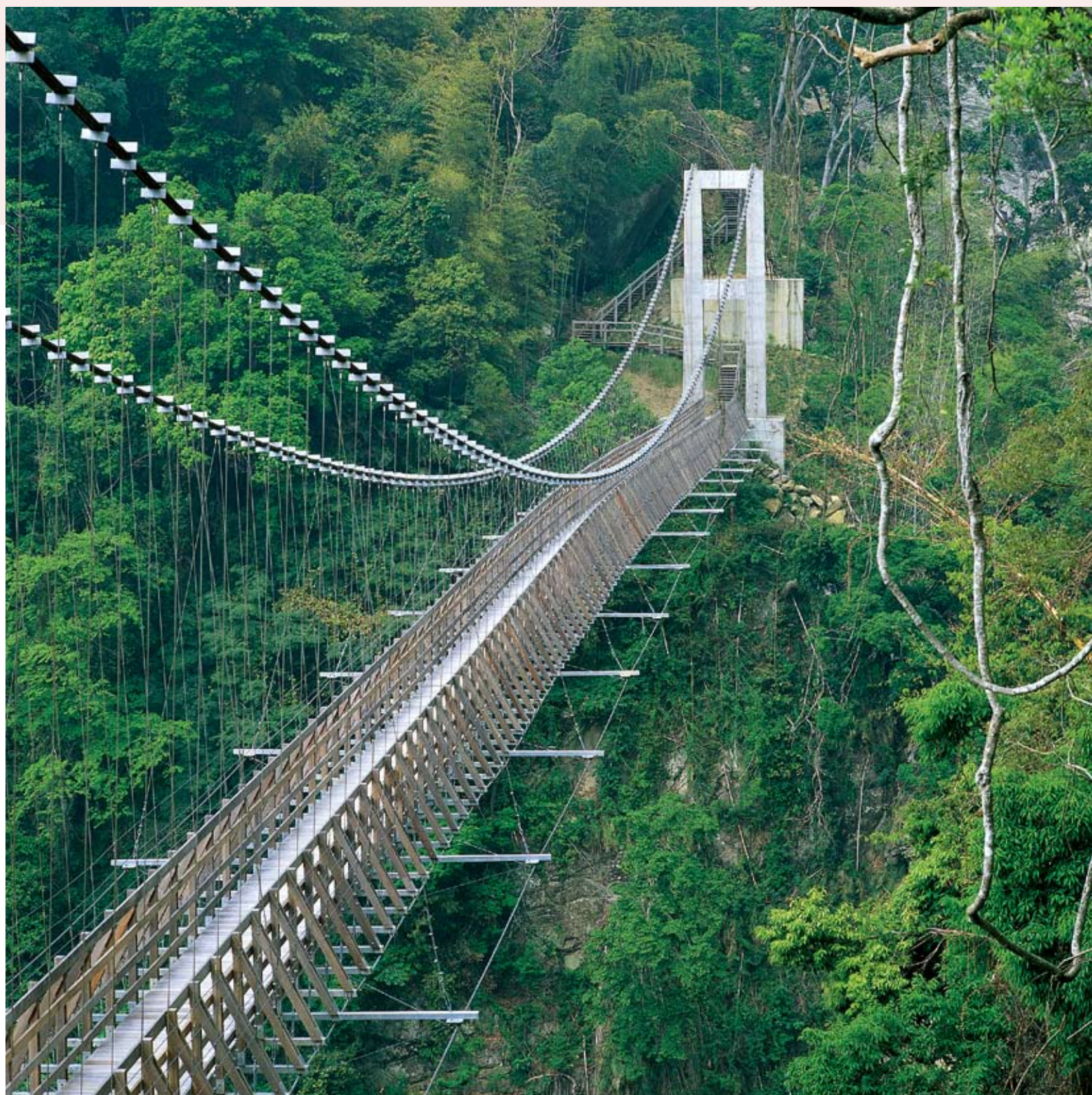
豐山·石盤谷吊橋 Shrpangu suspension bridge, Fengshan
